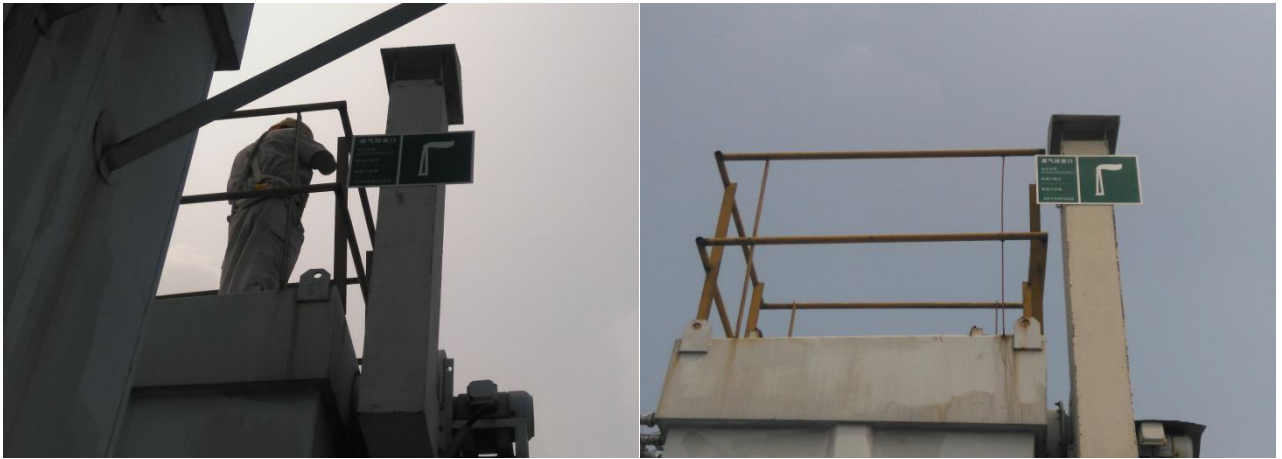
硅灰料仓除尘器排气筒 P3 粉煤灰料仓除尘器排气筒 P4
